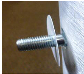
INCORRECTLY FITTED
